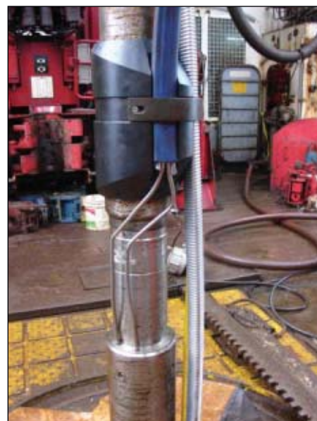
Rotating cable protectors shield the lines at the gas lift mandrel and downhole safety valve (Fig. 2).
